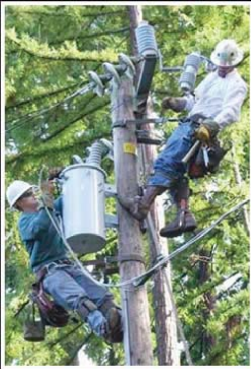
Following a lightning strike that knocked the old transformer out of service, Monterey general construction lineman Ronnie Laughlin (left) and lineman Jim Adams install a new 15-kilovolt unit to serve a Santa Cruz customer. December 2002.
